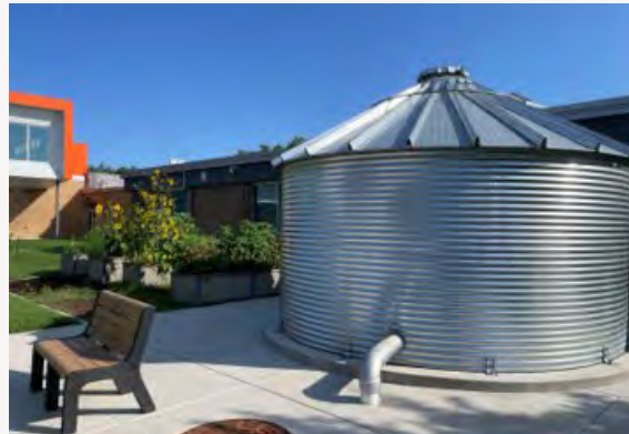
Norman Sims Park Cistern
