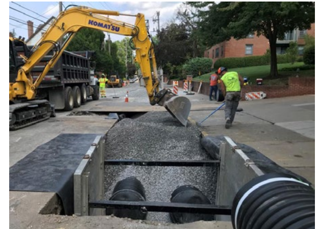
Construction of Maryland Avenue Stormwater Project in Shadyside (Credit: PGH2O)
