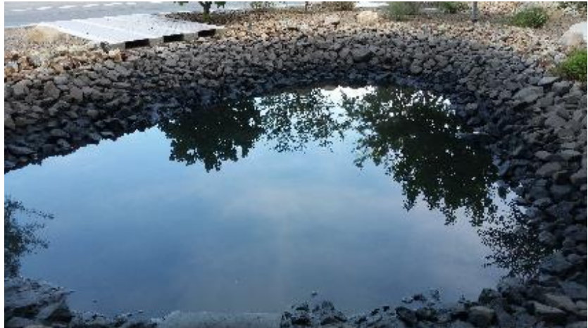
A rock lined basin with no sediment trap in Tucson holds water after a week after a rain event limiting the storage capacity of the basin and increasing the risk of mosquitoes.
